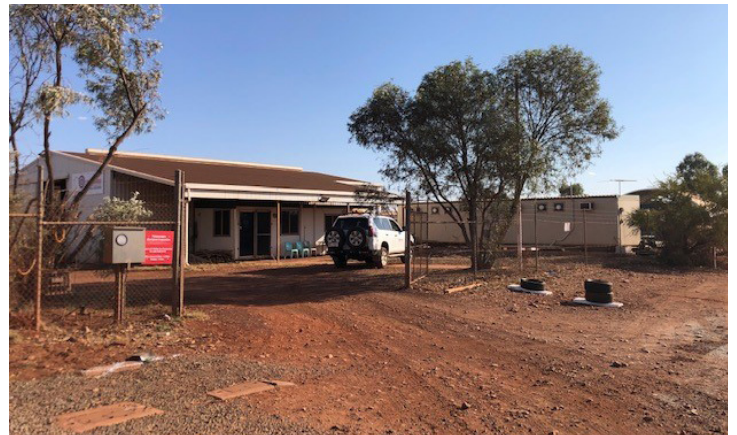
Ranger Program shed
